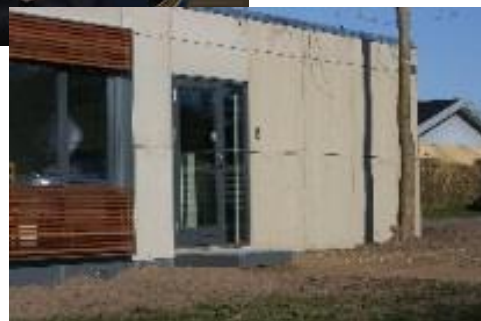
Addition building for bodyguards
